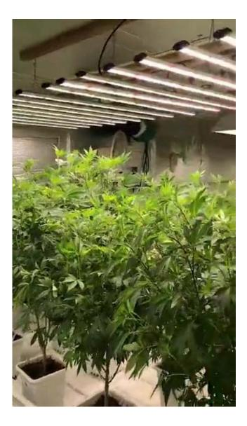
The IP65 rated, 240V AC, 200W GRP-240-200 grolux panel is supplied with a standard 1m suspension cable.
